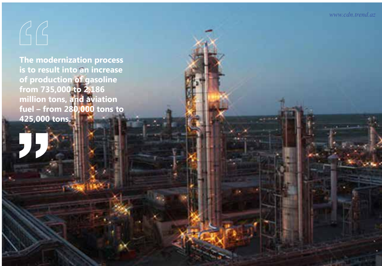
Modernization of the Shymkent oil refinery
